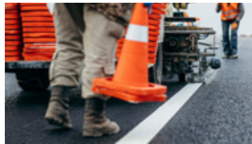
Construction and Installation
